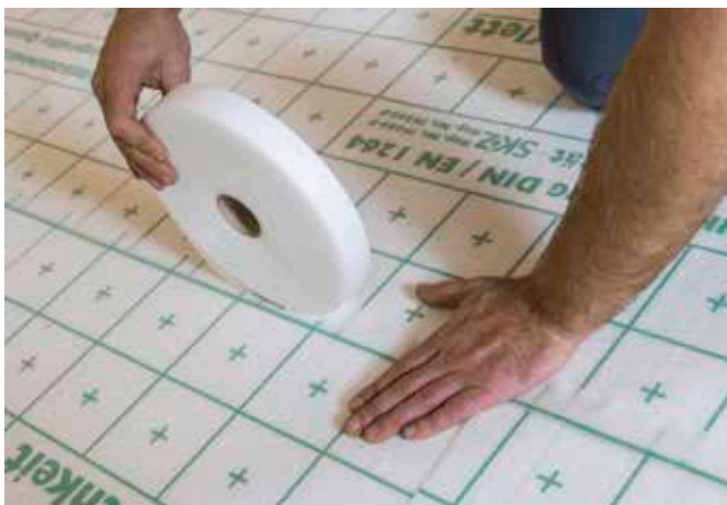
Once the EMPUR® hook and loop panels have been laid overlapping, the overhanging film is fixed to the connecting panel with connecting tape.
